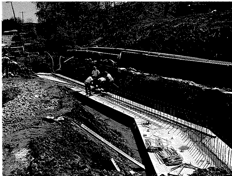
North Culvert Footer complete
