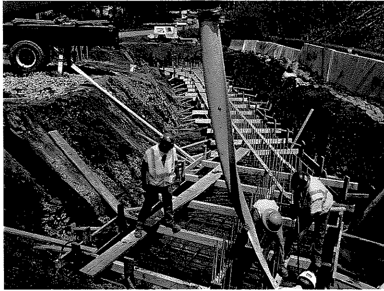
Concrete Placement in the North Foundation of the Duck Hollow Culvert
